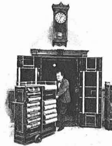
VAULT ENTRANCE ON MAIN FLOOR.
