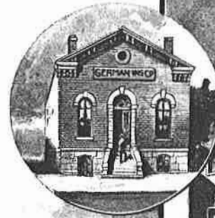
ORIGINAL OFFICE BUILDING.
