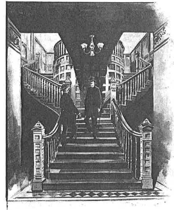
MAIN STAIRWAY TO OFFICE.
